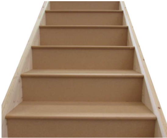
MDF Type 1A Carpet grade to stringers, treads and riser.
